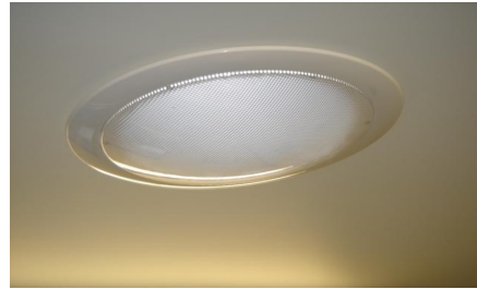
Ability to close diffuser for heat loss and operations in cooler climate zones
